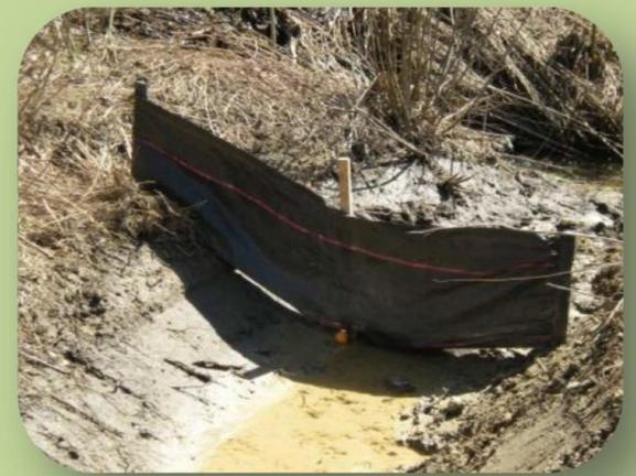
***WRONG!*** An example of an ineffective erosion control practice – silt fencing should be buried to a depth of about 8 inches and should not be used in drainage ways
