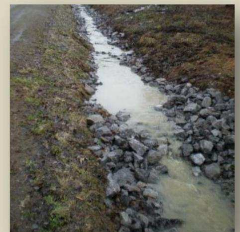
*Rock-lined ditches and check-dams are a cost-effective technique for reducing runoff from roads and ditches*
