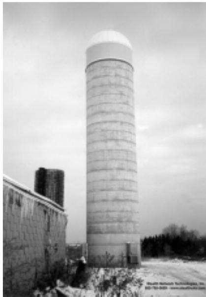
structures are uncommon, new "stealth" structures can be sometimes be built on which to mount the antennas. Rooftop sites with facade coverings, church steeples, farm-like silo sites with hidden antennas, flagpoles with flush-mounted antennas and fake trees with the antennas camouflaged by the artificial leaves are just some of the creative possibilities for making cellular antenna arrays "disappear".
