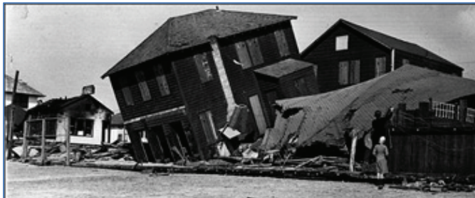
Long Beach lost many homes and other structures to the 1938 "Long Island Express." The potential for catastrophic losses among south shore communities has increased with rising seas and development in high-risk areas.
