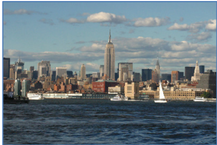
Infrastructure critical to both the state and national economies will be subjected to increased risk of coastal storm damage as sea level rises.
