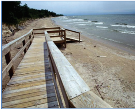
Beach erosion could lead to loss of recreational areas.
