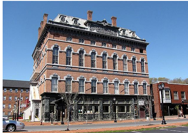
Figure 10. The Cohoes Music Hall is one of several properties located within the Study Area listed on the National Register of Historic Place
