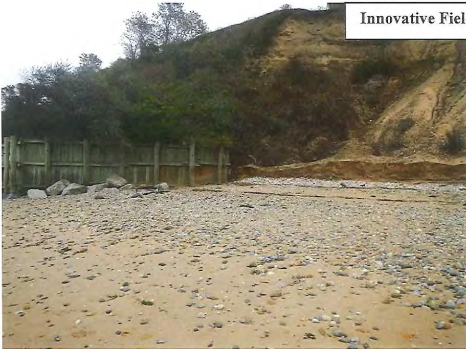
Photo 1 – View south along east side of eroded bluff
