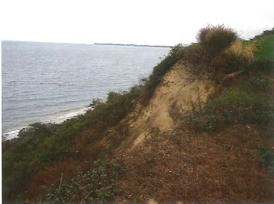
Photo 3 – View east along eroded top of bluff
