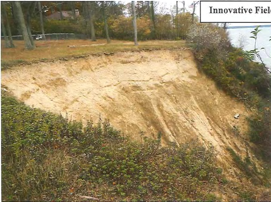
Photo 1 – View west along eroded bluff
