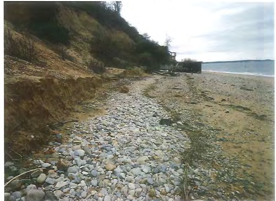
Photo 4 - View west along eroded shoreline and bluff
