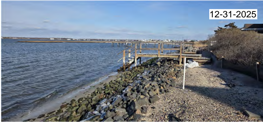
VIEW EAST: SHORELINE AT SUBJECT PROPERTY.
