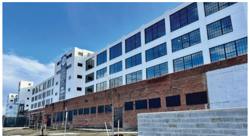
The former Endicott Johnson Shoe Corporation Victory Building (above), located in the Endicott-Johnson Industrial Spine BOA, has been transformed into a residential apartment complex (below).
